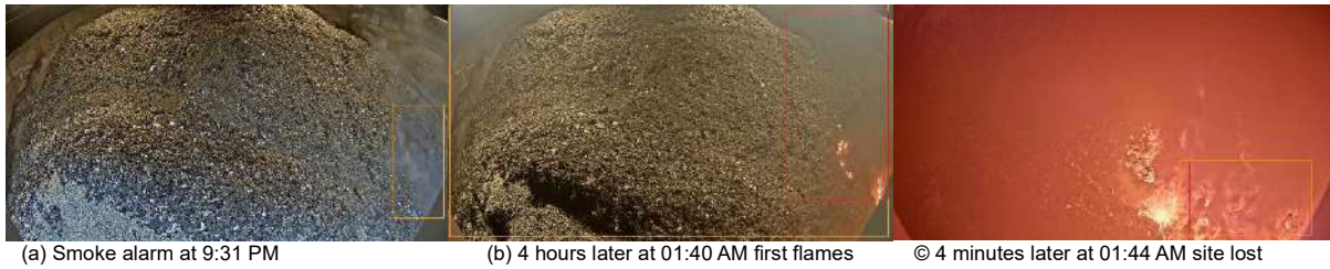
Figure 11. Example of a real incident with self-combustion in SRF waste storage.
